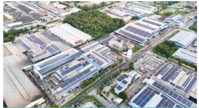
Solar Photovoltaic Rooftop Projects at LBA Beranang Factory
